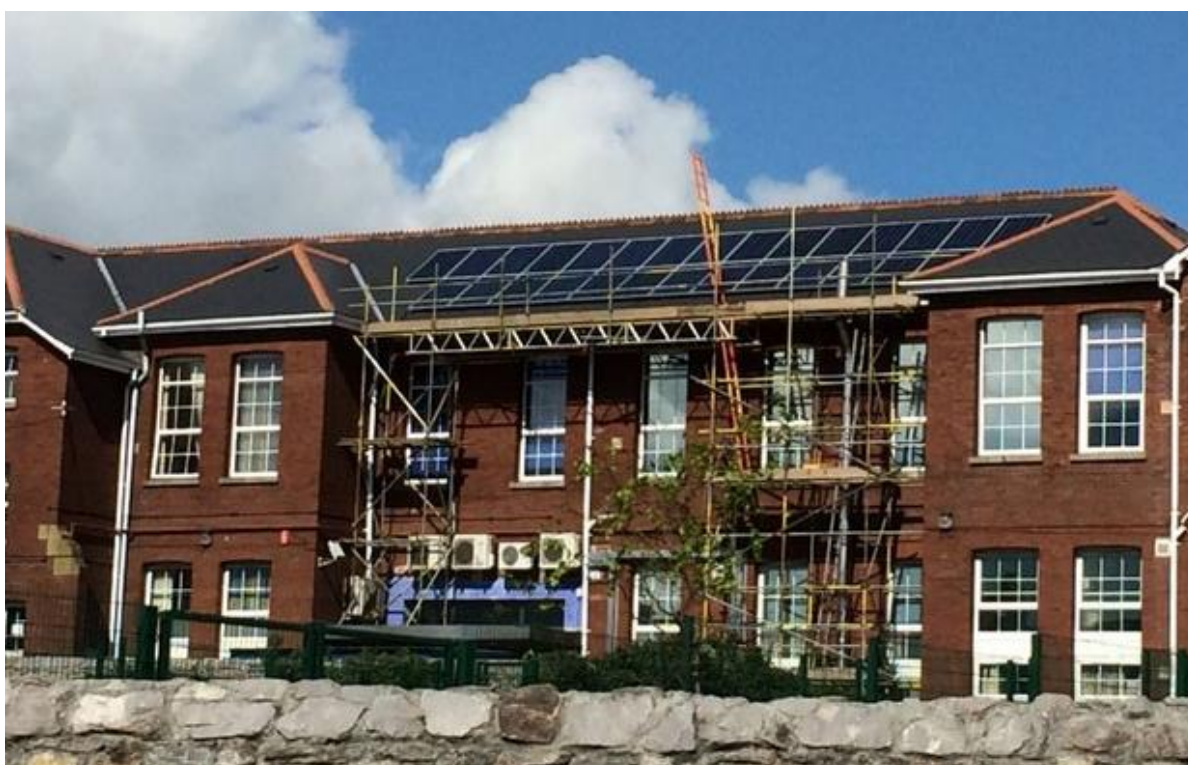
Solar PV being installed at Victoria Road School Easter 2014
